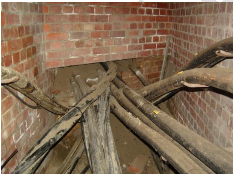
■ Figure 11 Substation Cable Exit Congestion – Wellington Street
